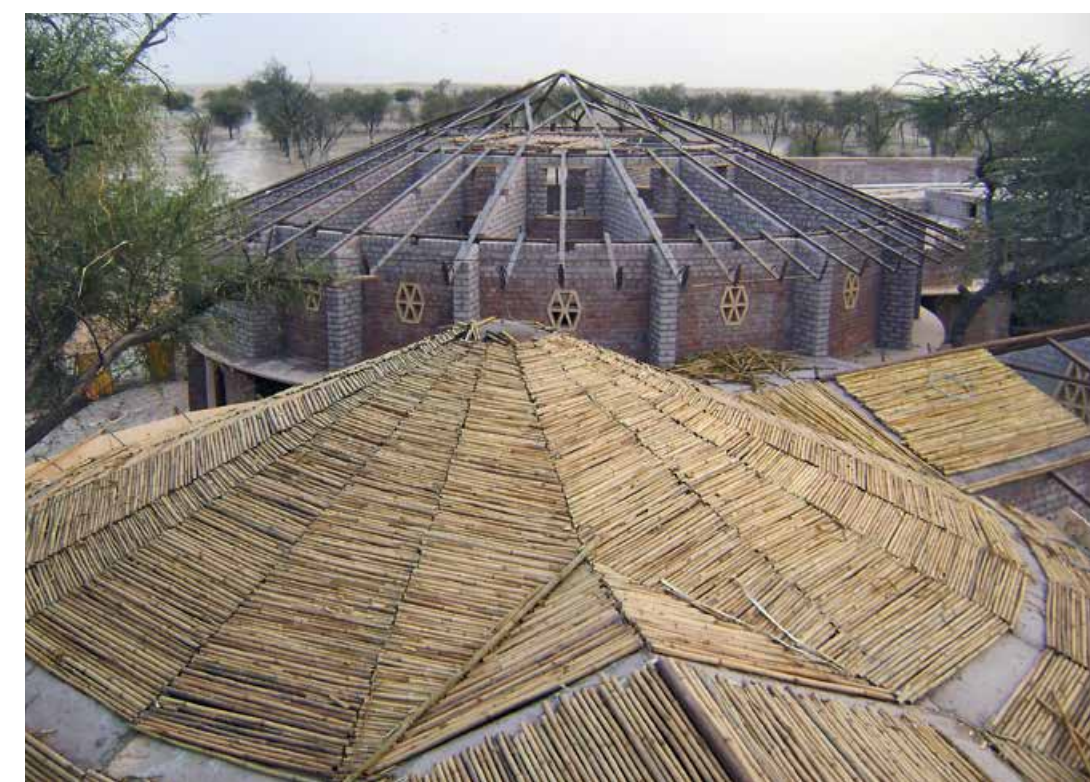
The 'neo-jhumpas' boast of an articulated triangulated steel frame that holds up a bamboo roof finally decked out in concrete. Above: A layer of soil and grass imparts thermal mass to the roof, thus lowering indoor temperatures
