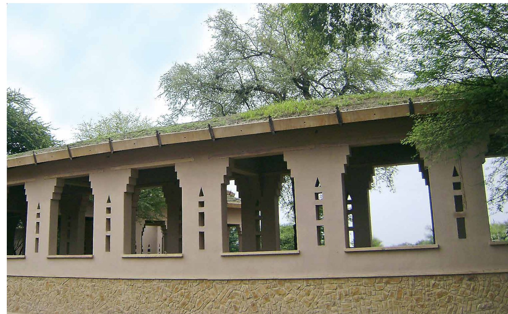
The 'neo-jhumpas' boast of an articulated triangulated steel frame that holds up a bamboo roof finally decked out in concrete. Above: A layer of soil and grass imparts thermal mass to the roof, thus lowering indoor temperatures
