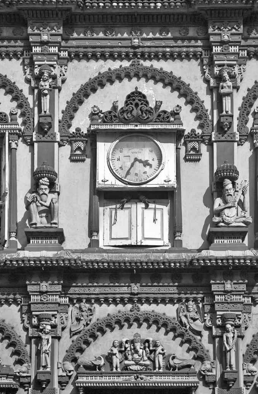
This page, Top: Dwarkadhish-temple@- Kalbadevi Below: Indian-Sailors- Home@-Masjid Opposite page: Keshavji- Nayak-Pyau-Clock- Tower@-Masjid-W
